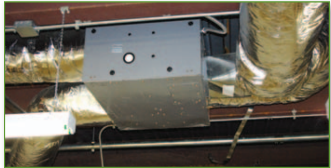
The low profile of the MV 750 makes for easy installation in tight spaces above the ceiling.
